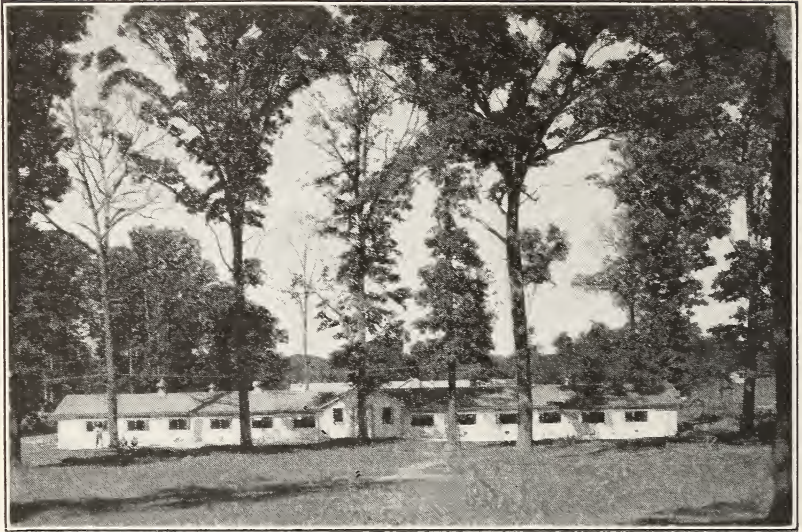
FIGURE 5.—One of the laying houses used in conducting nutrition investigations. Each wing is divided into six sections and the center part is equipped as a service room. The yards shown in front have concrete floors and the wire fencing extends over the top.
